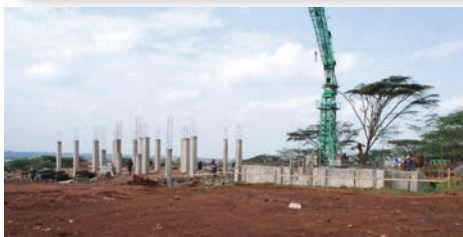
August 24, 2008 Judith Thomas Library Groundbreaking
